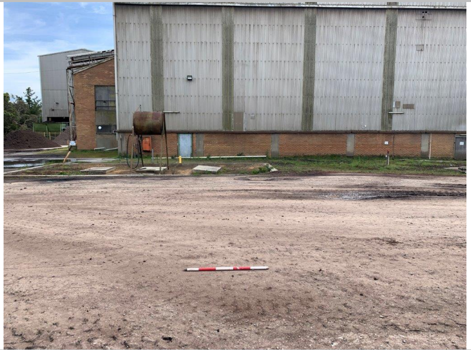
Plate 5: View of gravel pad (Matthew Barker 8/10/21), facing north
