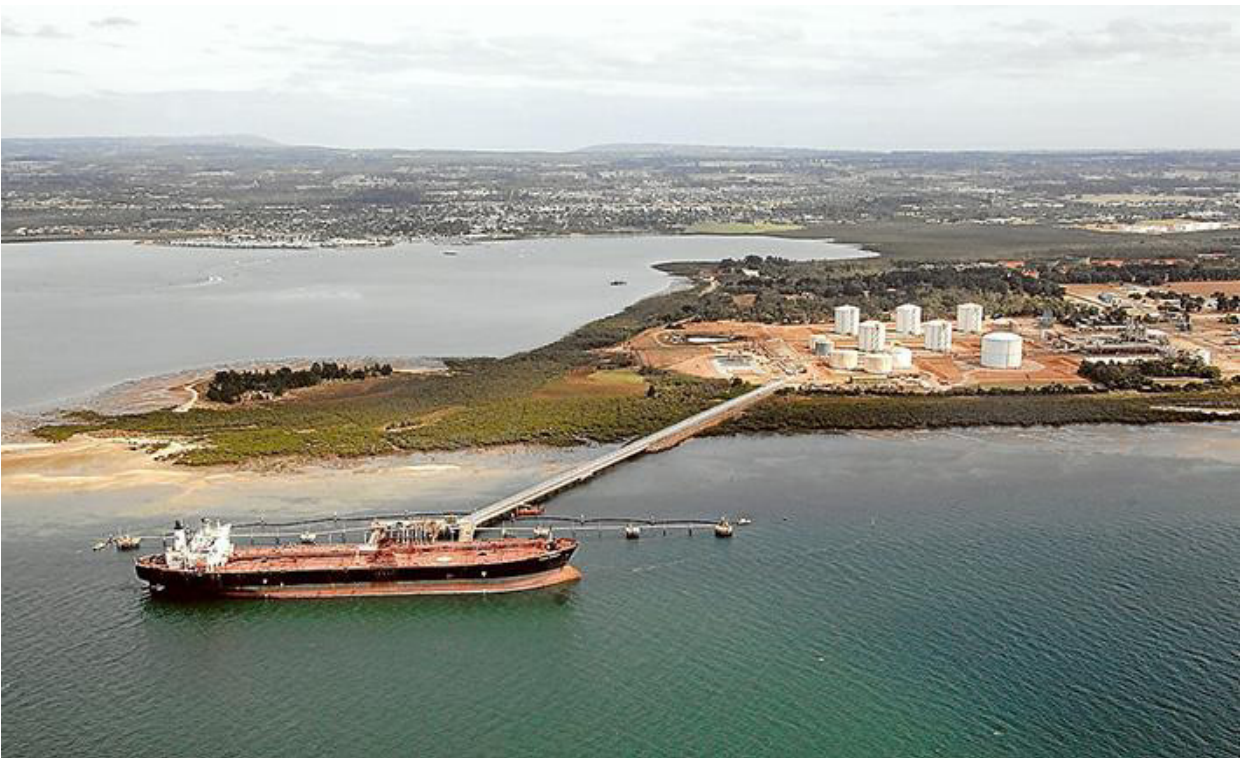
Long Island Point, Hastings
