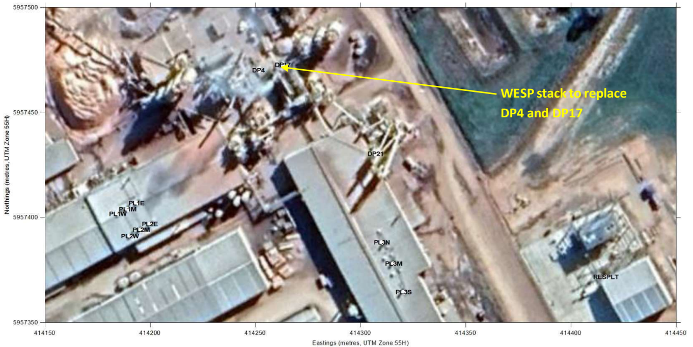
Figure 2: Aerial image of the location of the site licenced discharge points with assessed emissions and the plan as detailed in EPA Licence 9379.
