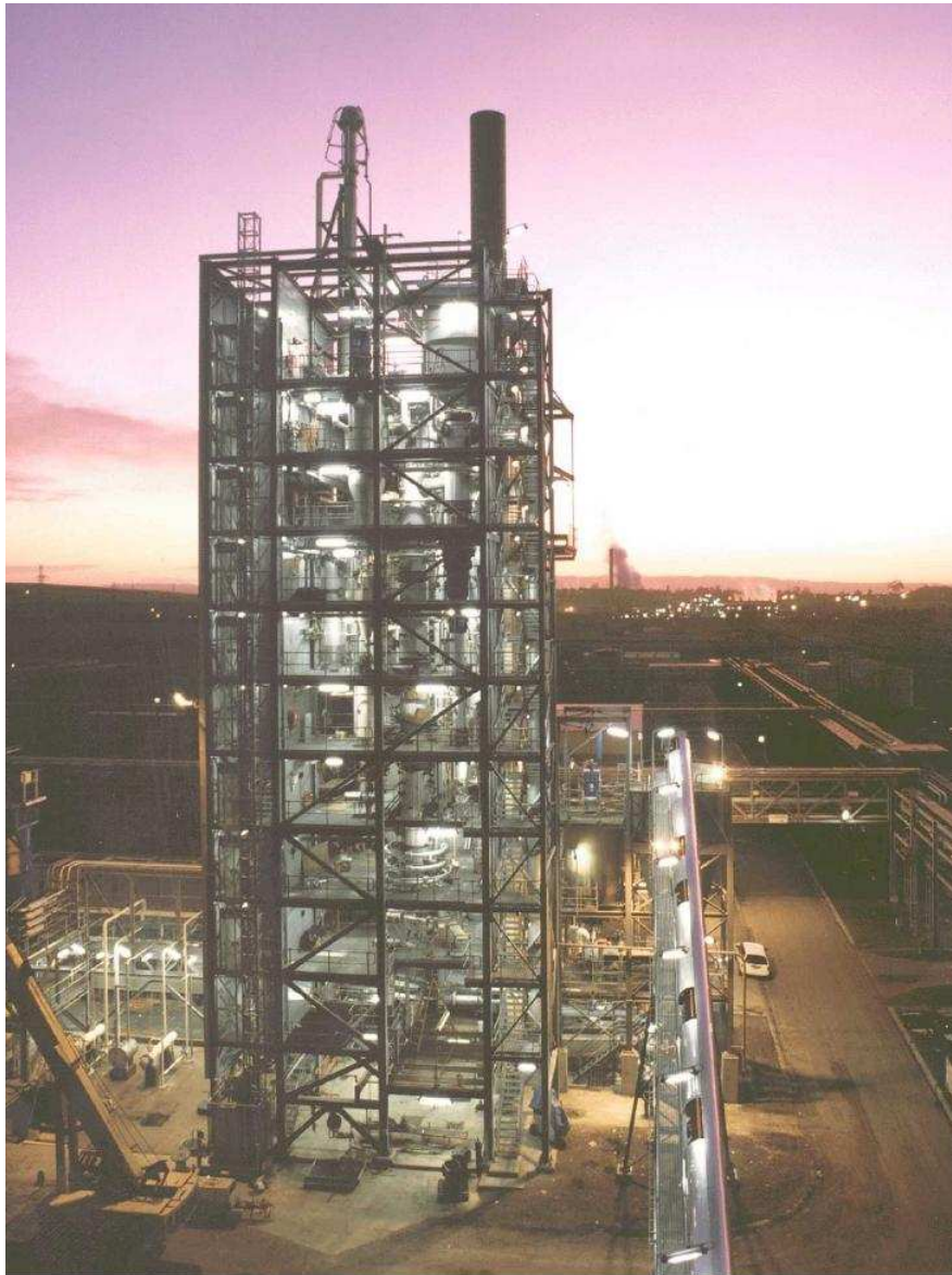
Figure 2 : Coal Gasification Development Facility (CGDF)
