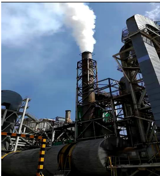
改造前 Before upgrading work
