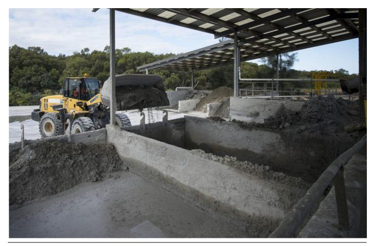
Figure 10. Washout pits being emptied. Source: Cement Concrete and Aggregates Australia (CCAA).
