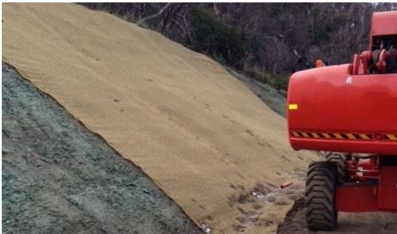
Figure 5.1. Slope stabilisation controls (photo courtesy of Regional Roads Victoria).
