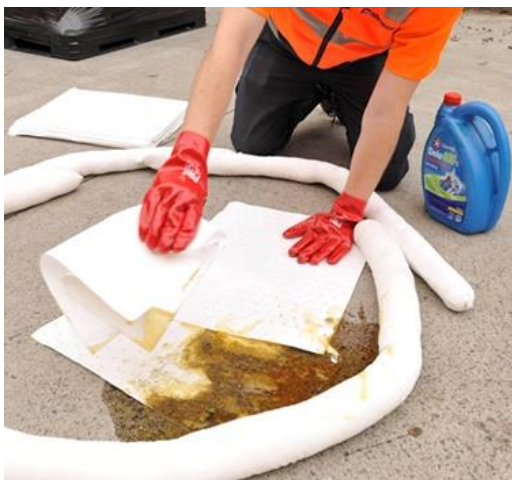
Figure 7.4. Containment and cleanup of a spill.
