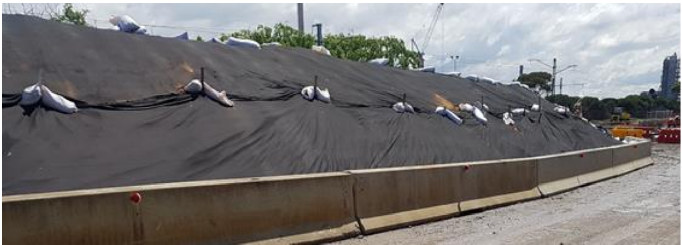
Figure 2. Covered stockpile (photo courtesy of McConnell Dowell).
