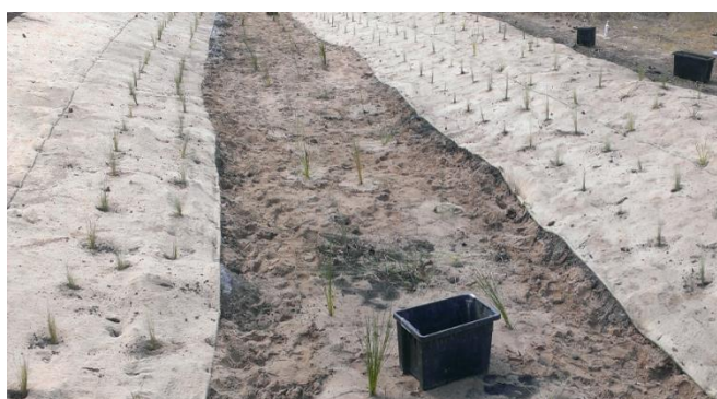
Figure 1. Swale under construction. (Photo courtesy of Fulton Hogan.)
