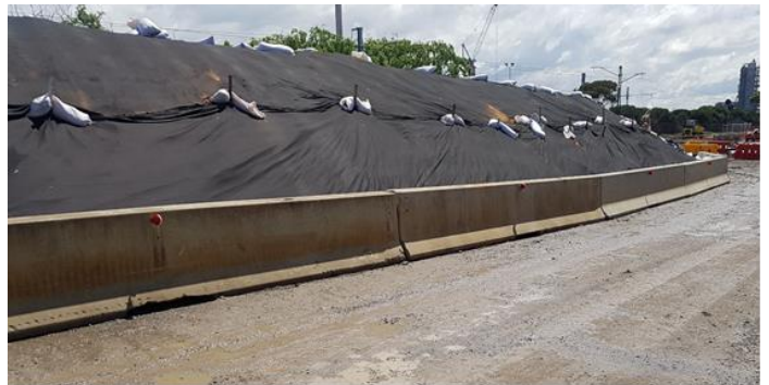
Figure 1. Covered stockpile. (Photo courtesy of McConnell Dowell.)
