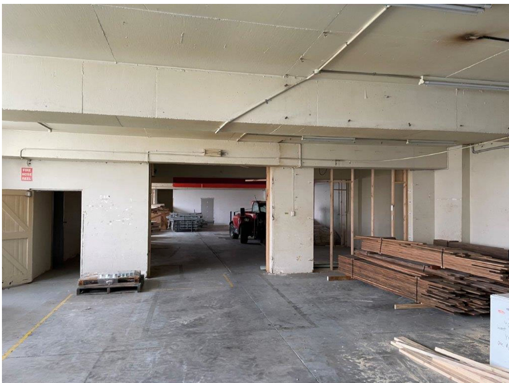
Inside 215 Albion St, facing south
