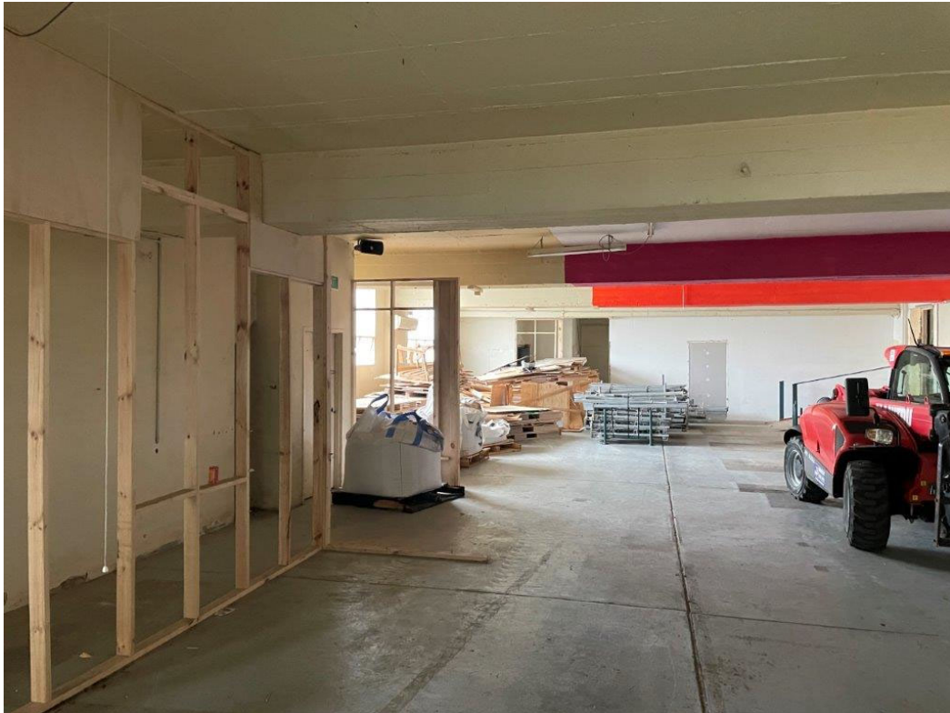
Inside 215 Albion St, facing south
