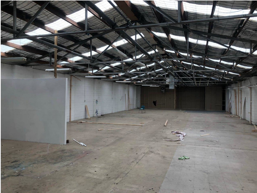
Inside 217 Albion St, facing south
