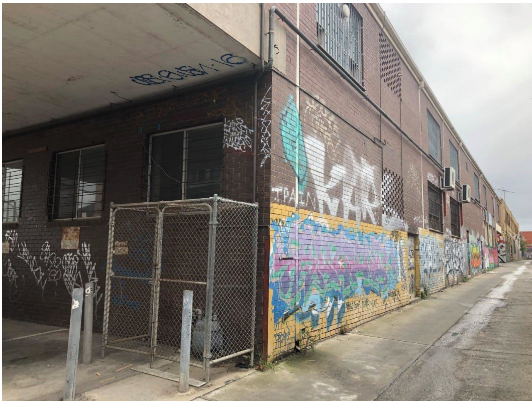
Exterior of 215 Albion St, facing north
