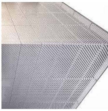
Image 5 Screen Perforated metal screen, fixed to metal sub-frame All in Colorbond Woodland Grey finish
