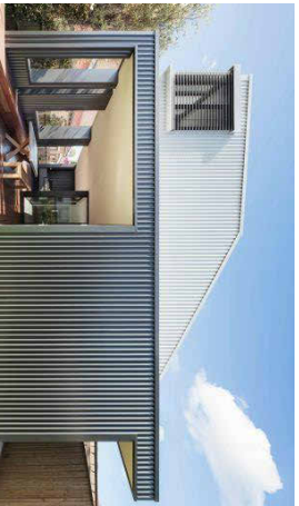
Image 2 Wall Cladding Colourbond Custom Orb - Woodland Grey Roof Cladding Colourbond Custom Orb - Slate Grey
