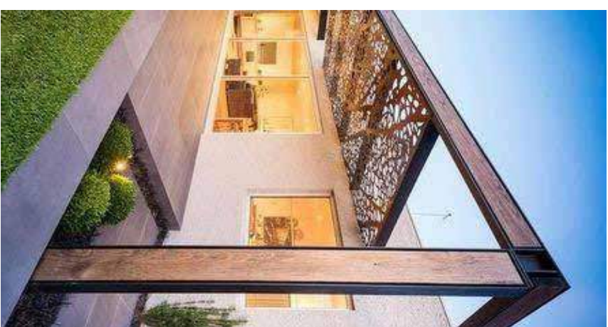
Image 5 Playground Columns Steel UC columns with timber inserts
