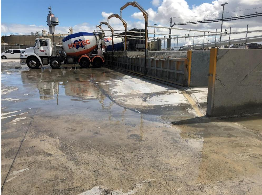
**Photo 23. Water being added to a cement truck within a dedicated bay at 32 South Wharf.**
