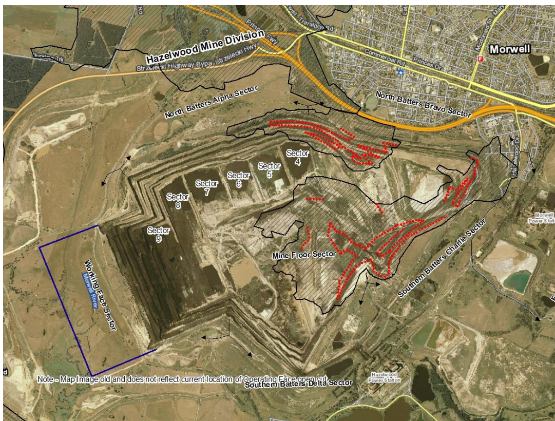
Figure 3 Map of the Hazelwood mine. Red colour indicates the batters on fire.
