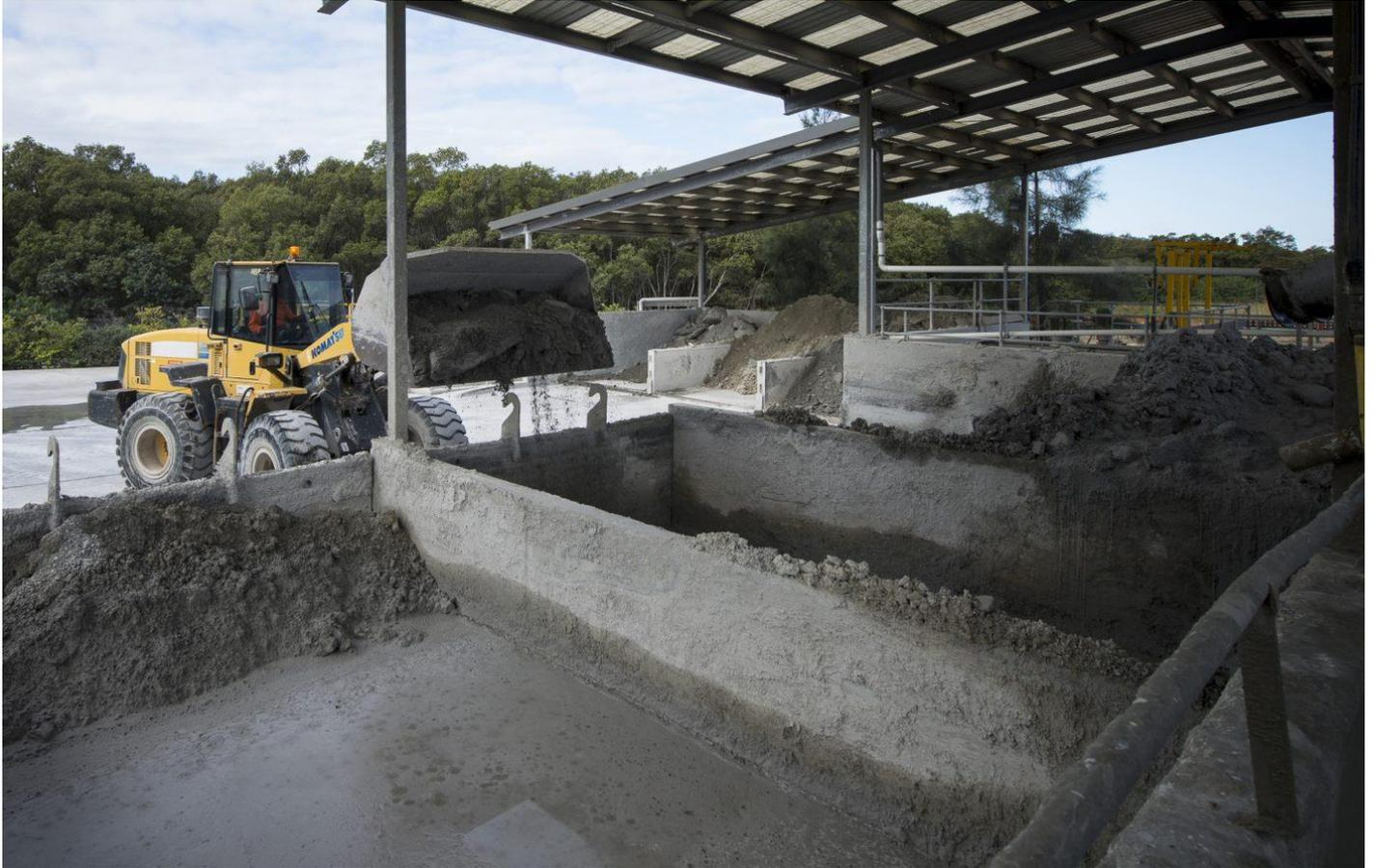
**Figure 10.** Washout pits being emptied. *Source: Cement Concrete and Aggregates Australia (CCAA).*
