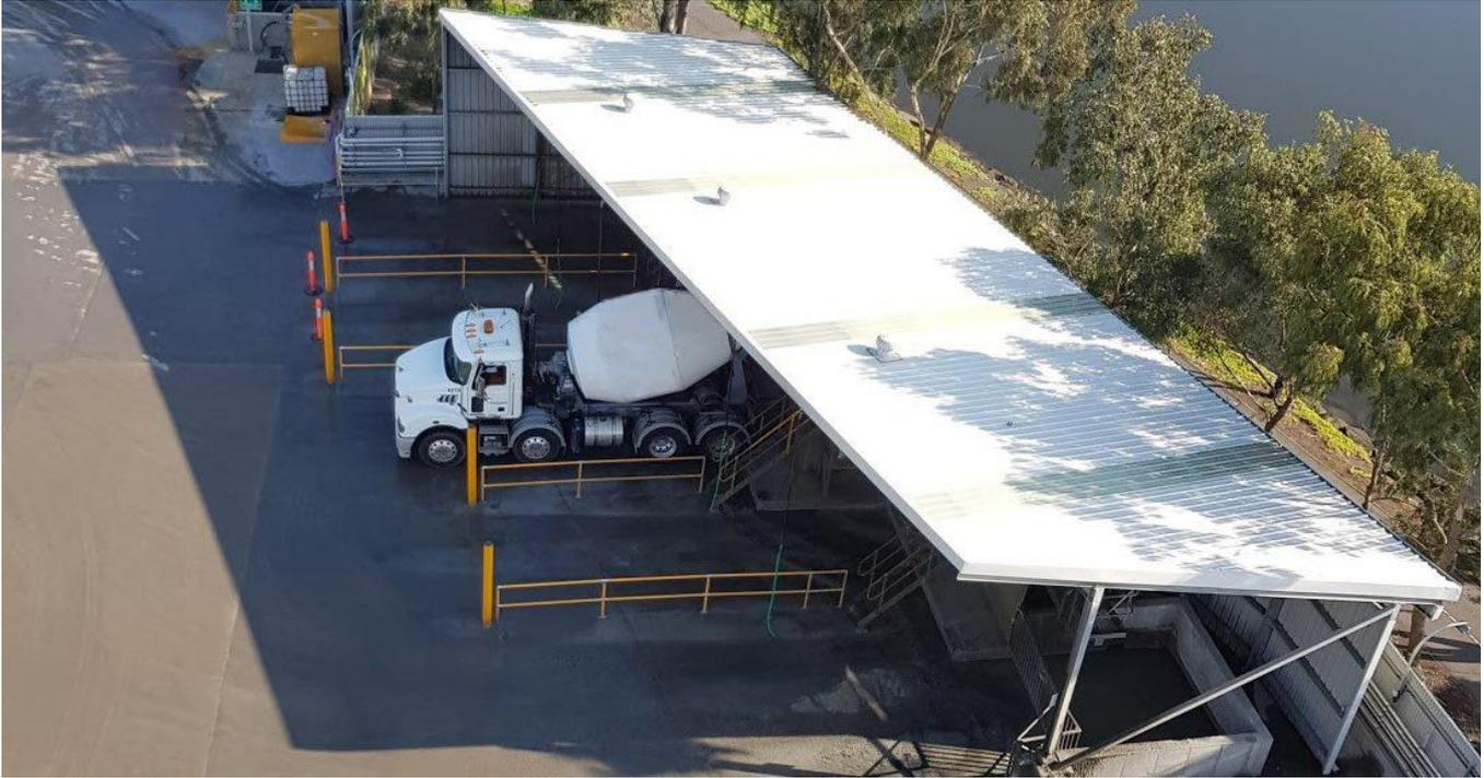
**Figure 5.** Roofed truck washout station. *Source: Cement Concrete and Aggregates Australia (CCA).*
