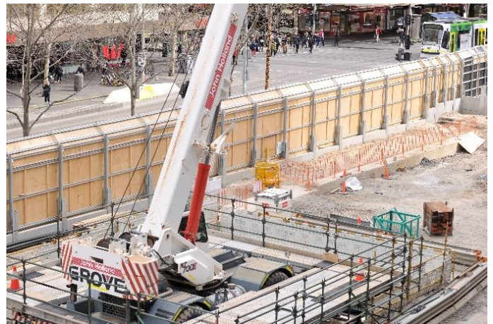
Figure 2. A temporary noise barrier erected around construction machinery to shield foot traffic from excess noise.
