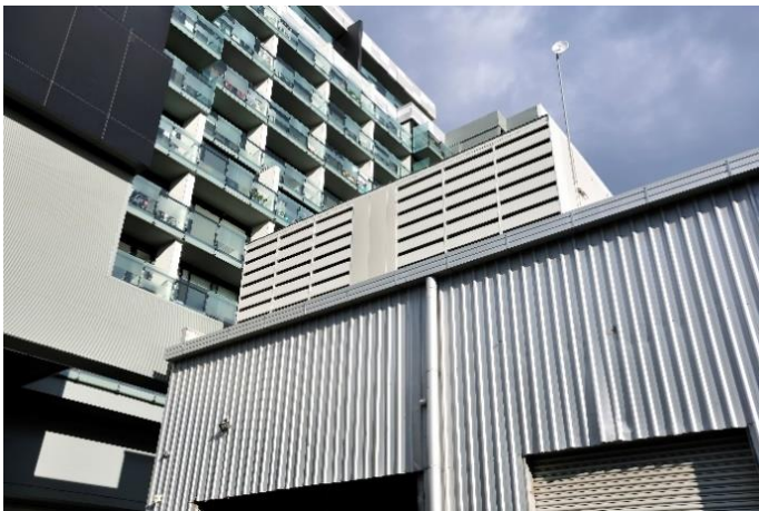
Figure 1. A full noise enclosure with acoustic louvres around ventilation system machinery.
