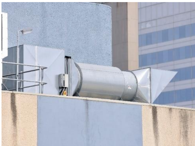
Figure 1. A circular attenuator on a rooftop.
