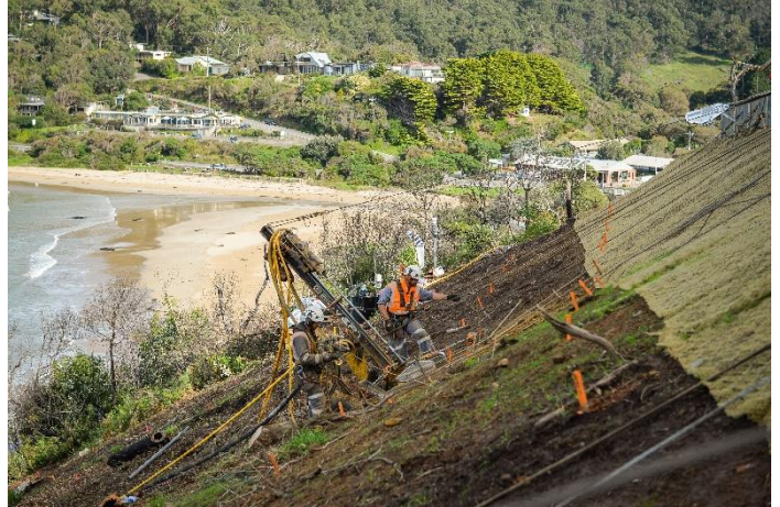
Figure 2. Slope stabilisation works. (Photo courtesy of Regional Roads Victoria.)
