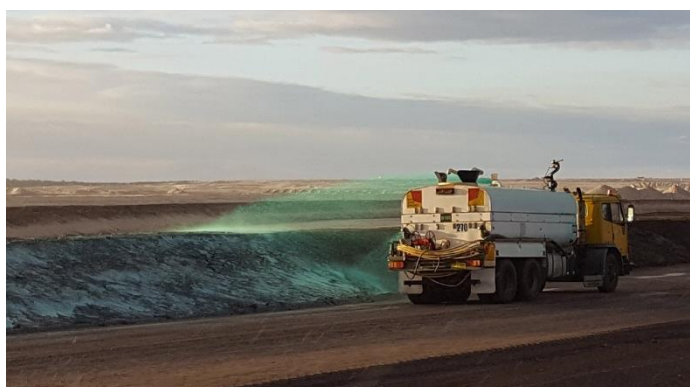
Figure 1. Water cart applying a soil binder/tackifier. (Photo courtesy of McConnell Dowell.)
