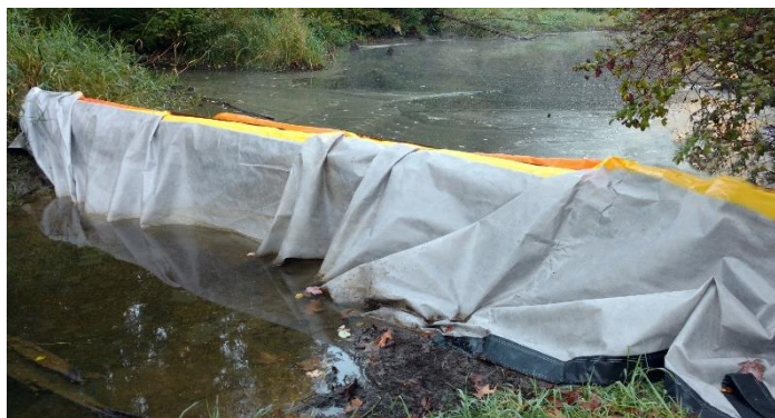
Figure 1. Engineered silt curtain installed to prevent migration of sediment for construction works within a waterway.
