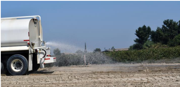
Figure 1. Water truck used on a dirt road to suppress dust.
