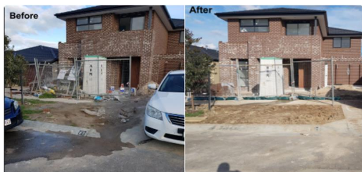
Figure 12: Stormwater issues from a construction site Photo: OPE program, EPA
