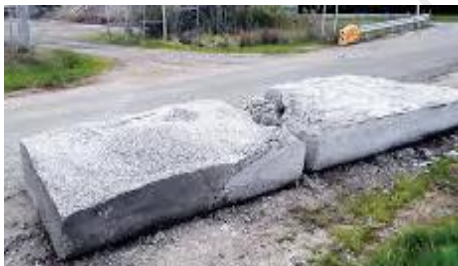
Figure 9. Dumped concrete. Photo: EPA
