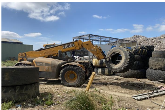
About 70 large tyres have been removed from the site
