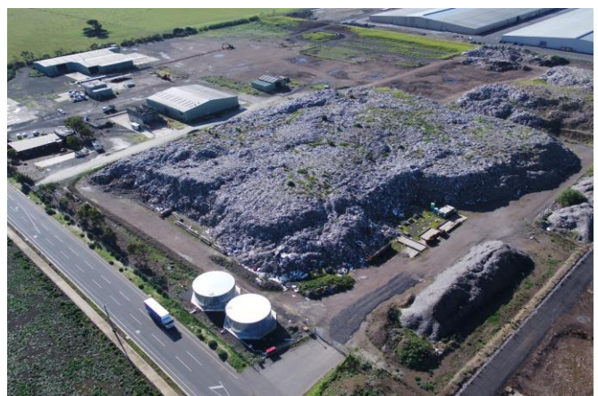
The Broderick Road site in April 2020, before the start of stage three clean up works
