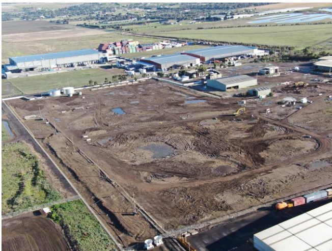
The Broderick Road site in June 2022, with all waste removed
