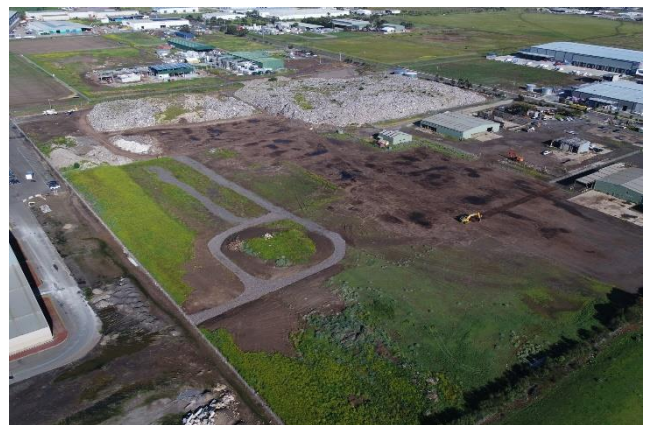
The Broderick Road site in April 2020, after the removal of 26,600m 3 of timber and 7,600m 3 of soil
