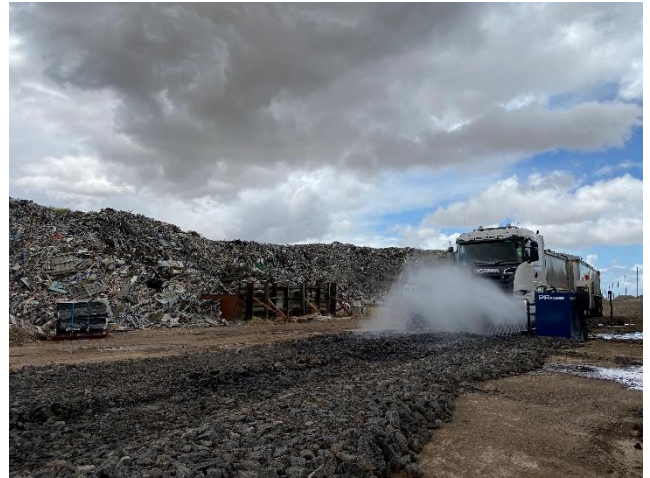
A wheel wash system helped reduce offsite impacts
