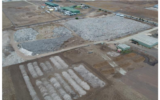
The Broderick Road site in April 2019, before the clean up started
