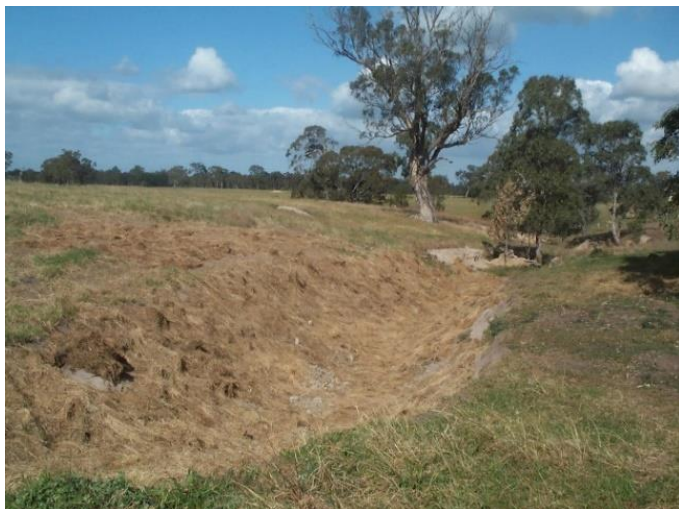
After: Cleared area ready for revegetation.
