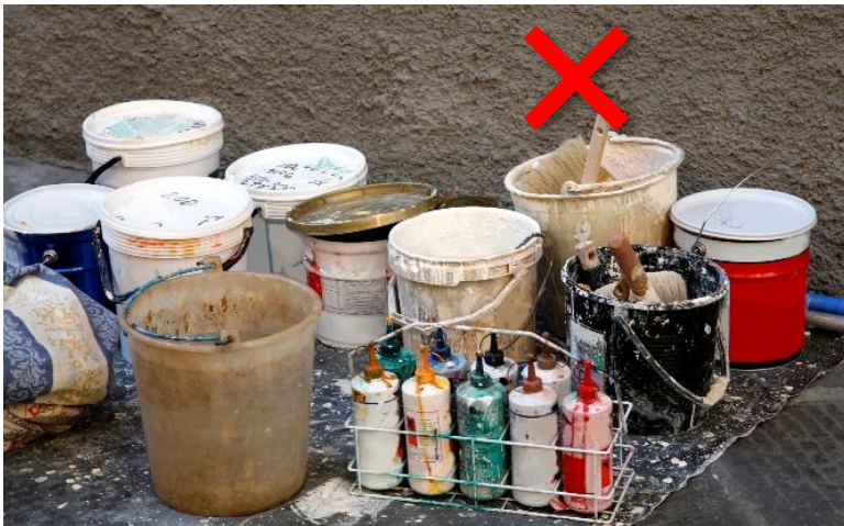
Figure 7.1. Incorrect chemical storage onsite.
