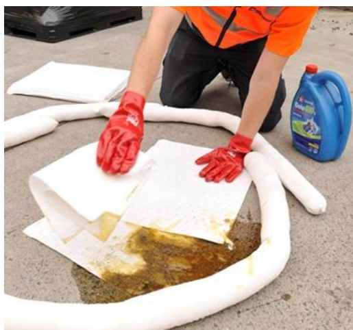
Figure 7.4. Containment and cleanup of a spill.
