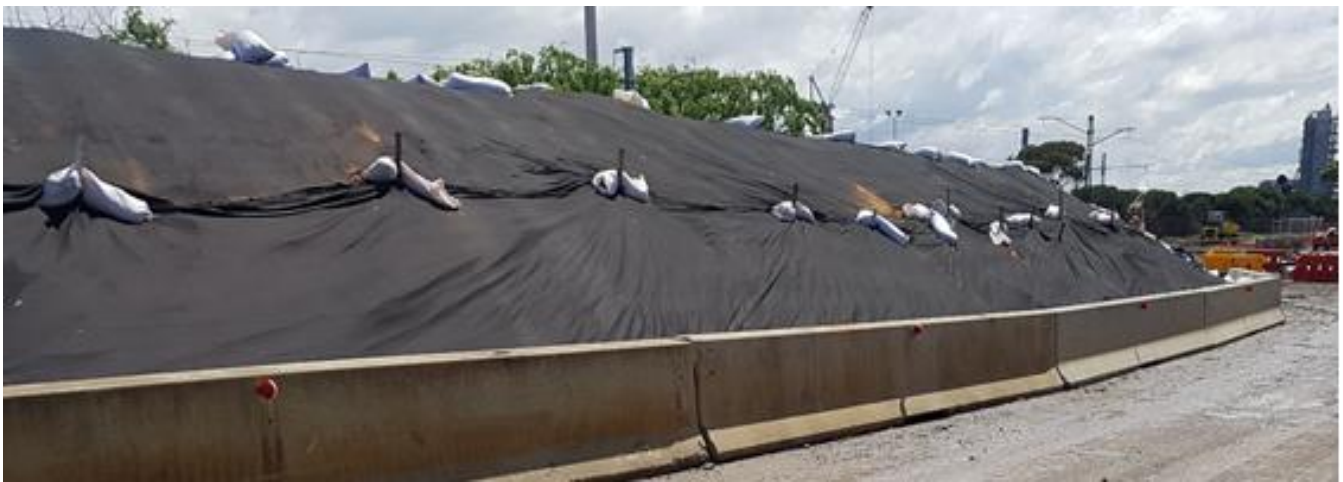
Figure 2. Covered stockpile (photo courtesy of McConnell Dowell).
