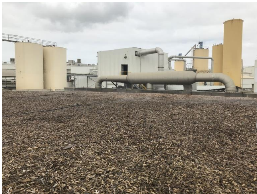
Figure 1: Open bed biofilter with vertical plenum inlet to two cells
